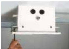
Adjust to ensure ceiling integrity
